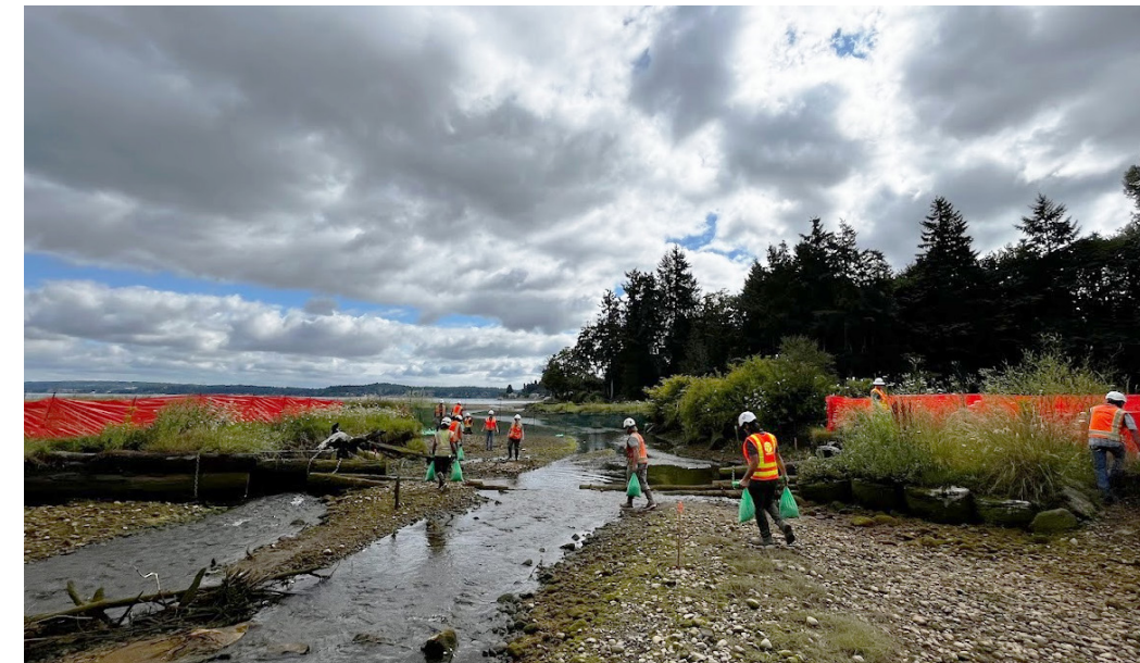
The project team uses block nets to prevent movement of fish into the work area.
